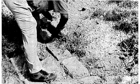
Figure 4. Setting mudbrick in erosion channel 3 (July 24, 1997).
